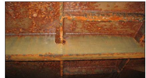
Figure 3.1.8: General breakdown of coating
