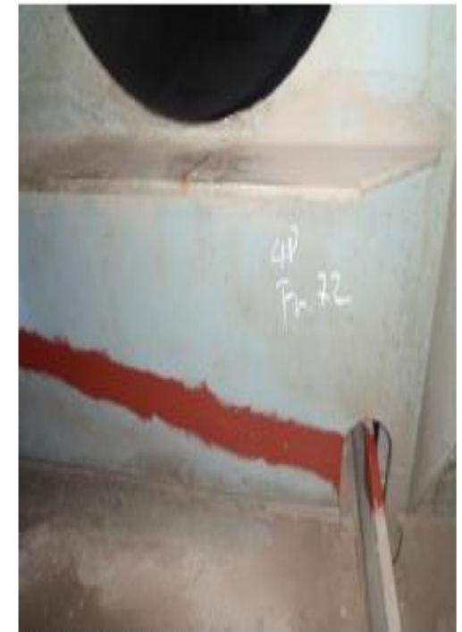
Crack on the web
